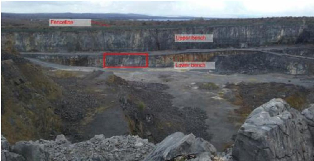
Some instability in the rock face is evident predominantly from blast damage during the operation of the quarry, with open discontinuities (joints and fractures), loose rock and the accumulation of debris resulting from spalling and failures present at the base of the lower and upper benches, see **Figure 3.5** below.
