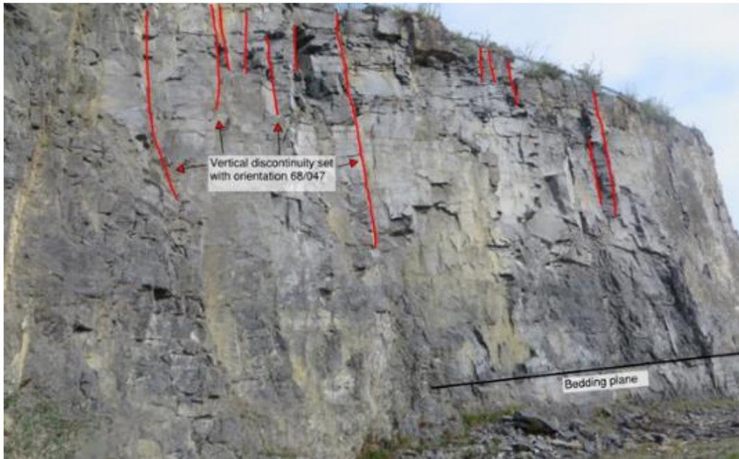
The vertical and horizontal discontinuities are visible on the exposed quarry face and are more evident in the upper bench wall, as the lower bench wall has been heavily affected by blast induced fractures.
