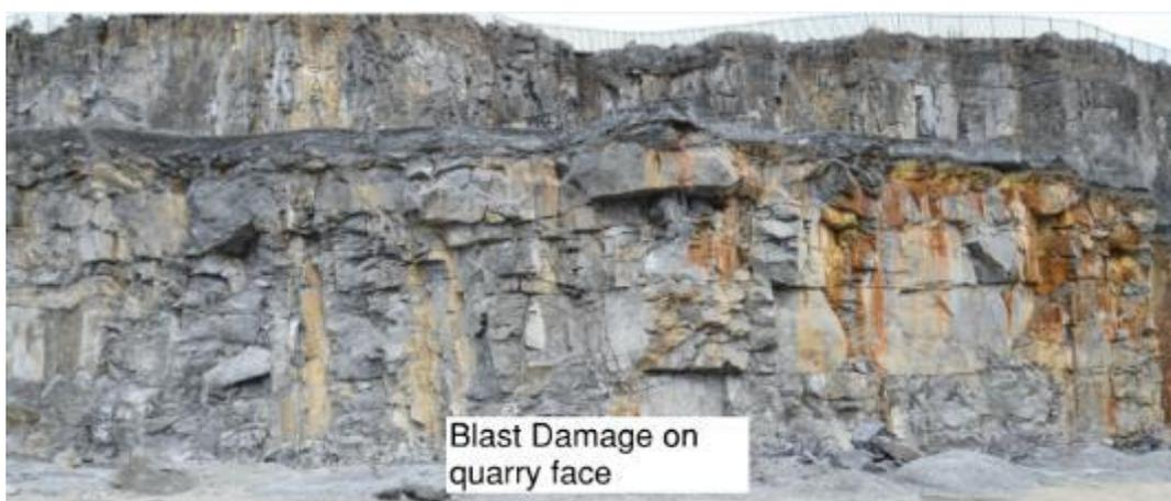
Given the nature of the fracturing and the evidence of failures, the angle at which the current rock face stands is too steep in parts, suggesting that this unprotected face, if left in its present state will continue to erode and may potentially impact the overlying Limestone pavement if a deep seated slope failure was to occur.
