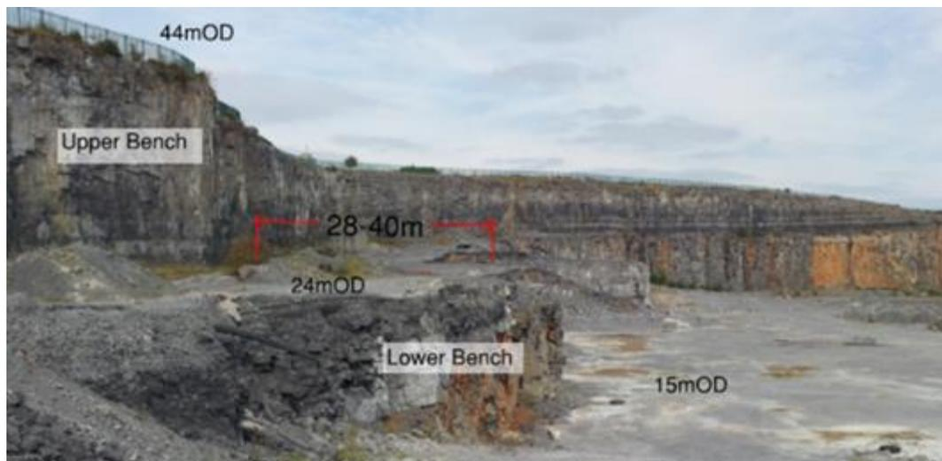
The quarry boundary is defined by a steel fence on a concrete plinth, which borders the Limestone pavement within the Lough Corrib cSAC. There is an average distance of approximately 1m between the edge of the fenceline plinth and the top of the upper quarry bench. **Figure 3.4** below shows a view of the western quarry wall from a distance, outlining the lower and upper bench and boundary fence.
